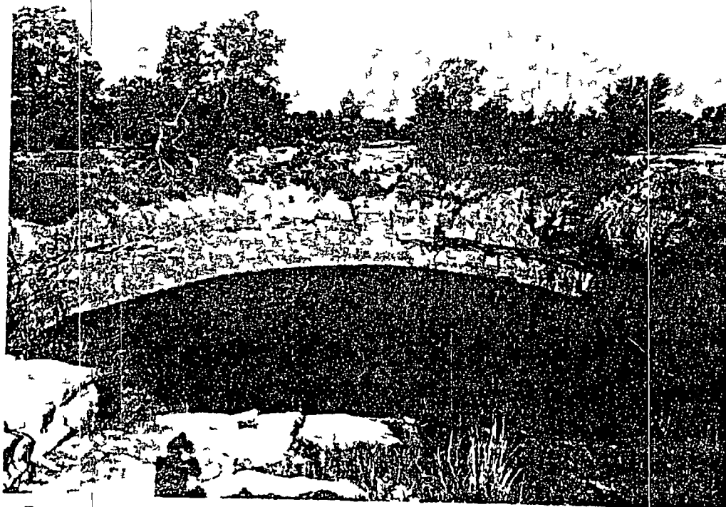
FIGURE 6 - Surface collapse 2 in sec 11 T 35S R 23E northwest of Treece Kansas
